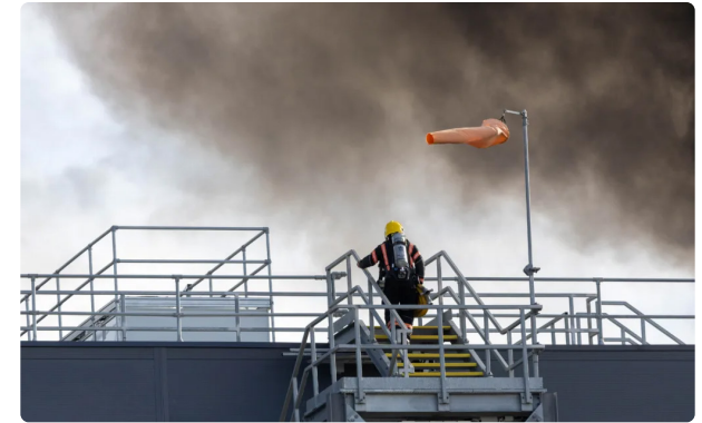
Solar panels catch fire at £70m Lidl distribution centre in Peterborough
